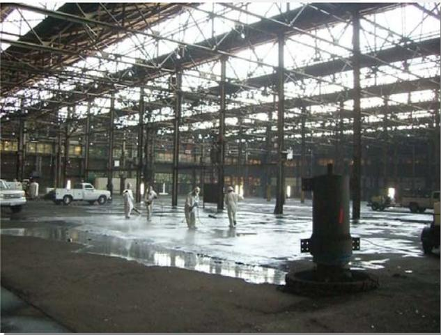
The removal of the roof ACMB was extremely challenging and required very stringent fall protection and material handling controls considering the workers were removing 500,000 SF from a sawtooth roof 60 ft in the air.
