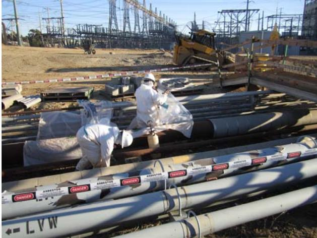
Once all the pipe coverings were removed, windows/drain on the pipes were opened with a non-sparking rivet buster tool to remove the contents and prevent spillage during the piping demolition. The contents were removed utilizing a vacuum truck when possible and transported to the tanks through existing access openings. The demolished pipes were transferred to the tanks for further processing.
